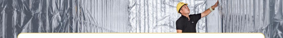
**DID YOU KNOW?** Thermal liners have been proven to reduce the risk of fire for self heating commodities such as charcoal. The phenomenon of self heating occurs when the substance is submitted to temperature increase and the availability of oxygen. By vacuuming most of the oxygen out of the MSC Thermal Liner combined with the reflective properties of the thermal liner, we significantly minimize the risk of self combustion and help reduce temperature fluctuations.
